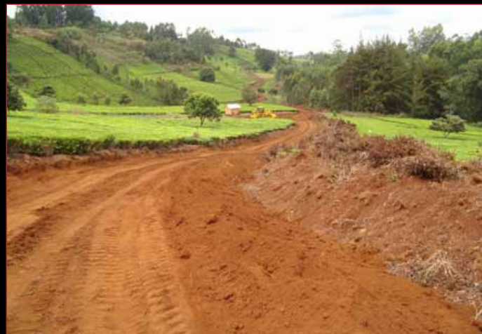
Proposed Access Road to Outfall portal site
